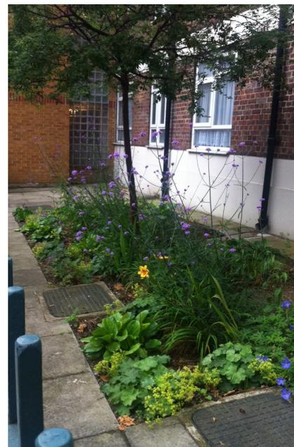
The next step is to consider the size of the rain garden. The bigger the rain garden the better. Experienced 'rain gardeners' in the US suggest that rain gardens are between 3m and 5m wide, with the length adjusted to suit the slope and area available. Although a rain garden of any size may bring some benefits, if it is very small, it may overflow too frequently and may become waterlogged and less effective in reducing run-off rates.
